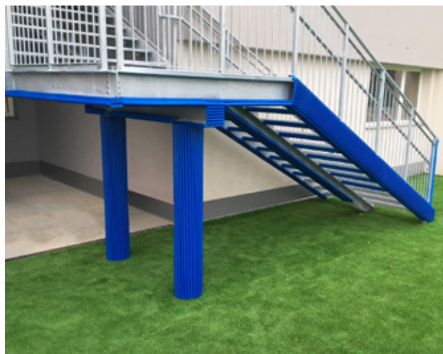
EMERGENCY STAIRWAY | ONDA 22 MM
